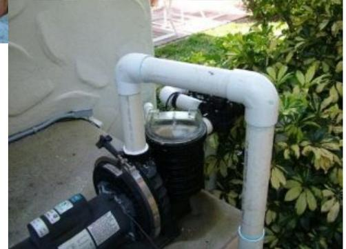
3.) Locate a space to mount the black flow-cell chamber. **Always install on the return line.** If possible, install the chamber after the filter, but it is not required if there is not enough space. If necessary, you can re-pipe an entire section to allow proper room for the electrode chamber or **ScaleBlaster** coil.
