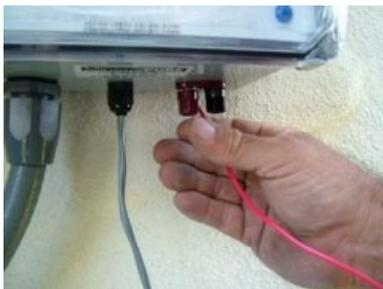
1.) Insert the pre-stripped end of the signal cable into one of the two binding posts located on the bottom of the control box. It does not matter if you hook it up to the red or the black binding post. The receptacle post can be unscrewed by turning it counter-clockwise. This will expose a small hole in the post. Tighten the receptacle post as much as possible with the signal cable completely threaded through the hole.
