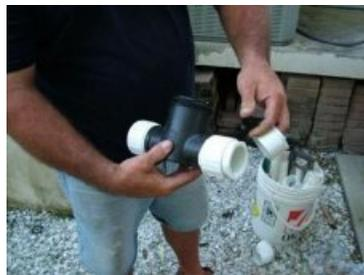
2.) If the pipe size where the flow-cell chamber is being installed is 1 1/2", glue the two reducer bushings (2" x 1 1/2") into the male adapters. This step is not necessary if installing on two-inch pipe.
